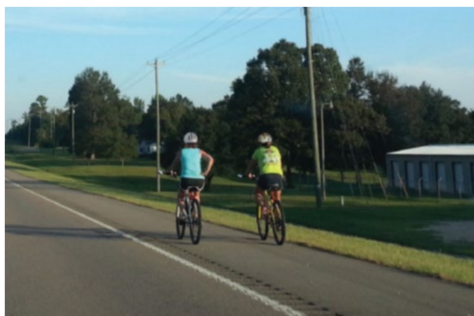
Figure 4.3 Bicyclists using a 4-foot paved shoulder with a rumble strip
